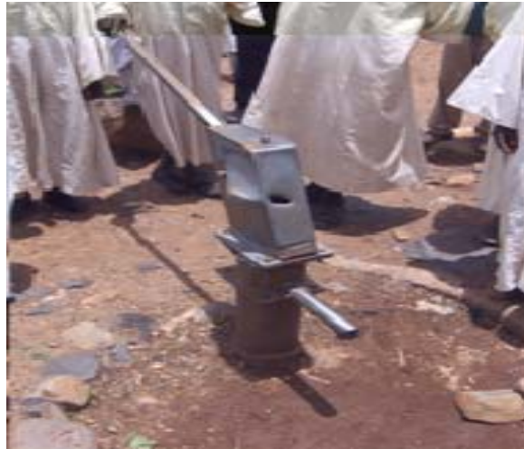
Photo 17 Water pump made inoperable by bomb shrapnel
