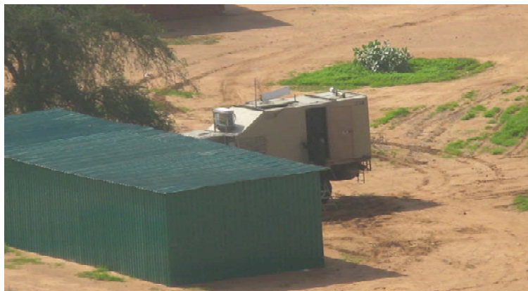
Photo 11 New hangar constructed and suspected unmanned aerial vehicle control vehicle, El Fasher airport, 11 August 2008
